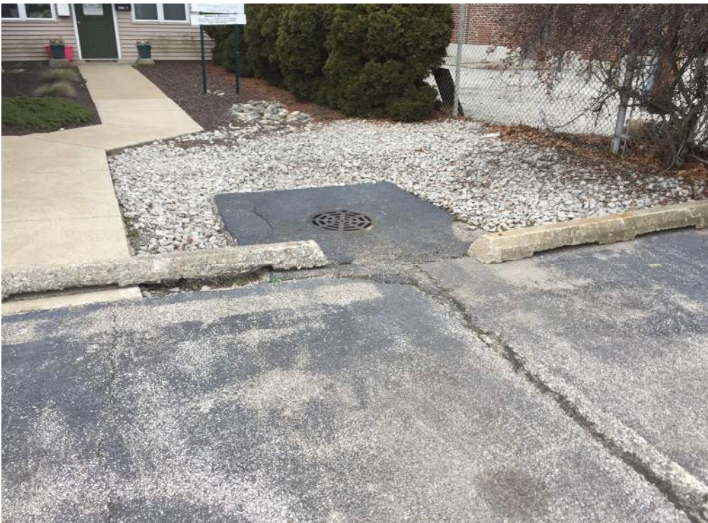
Photo 14: Stormwater drains on Subject Property
