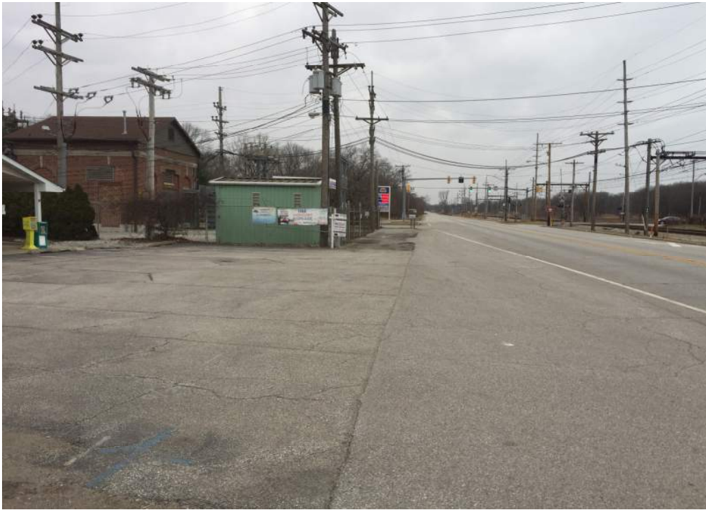
Photo 3: West adjacent property (electric substation, residential) facing west along Dunes Highway
